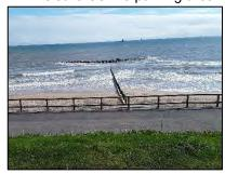
Photograph 11: Groynes and wooden posts along beach for support and protection
